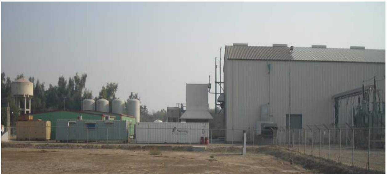
Two views of an installed power plant
